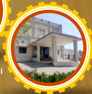
Bal Unit - 6 Udaipur API & Intermediate GMP Facility
