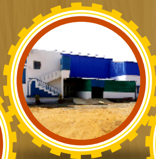
Bal Unit - 5 Sangli GMP Facility
