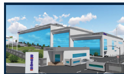
API Facility II PITHAMPUR, MADHYA PRADESH
