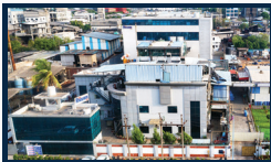
API Facility I ANKLESHWAR, GUJARAT
