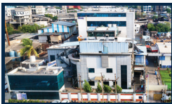
API Facility I ANKLESHWAR, GUJARAT
