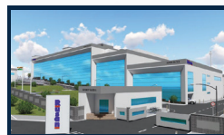
API Facility II PITHAMPUR, MADHYA PRADESH
