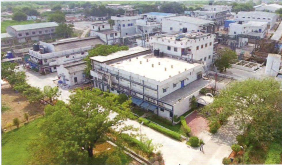
Unit-1-Deosugur, Raichur, India API Onco & non-Onco Facility. 7 API blocks with 325 KL capacity
