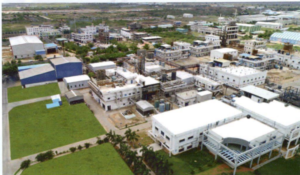
Unit-2-Chicksugur, Raichur, India API Onco & non-Onco Facility. 10 API blocks with 522 KL capacity
